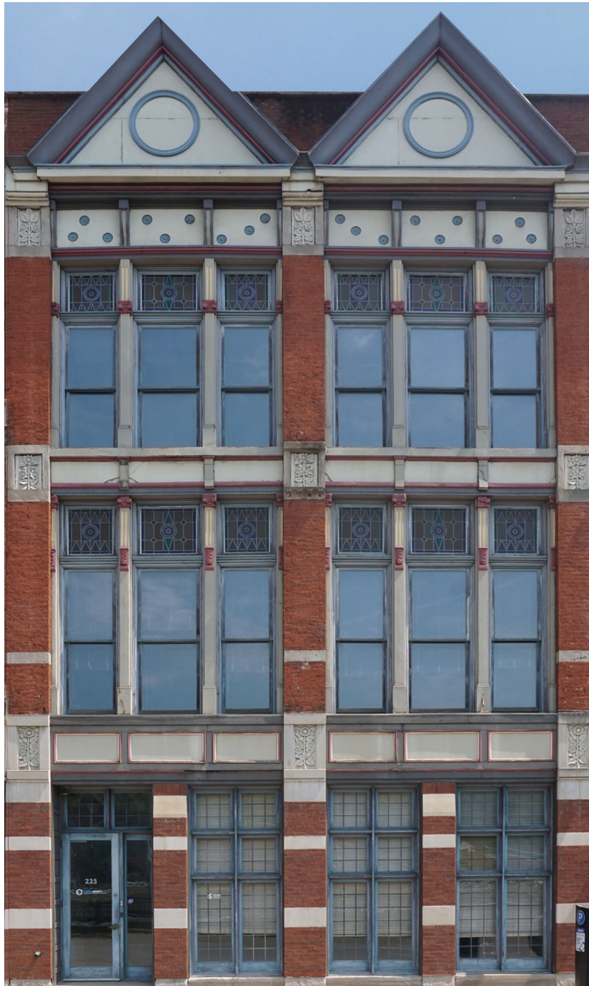
235 Fort Pitt Blvd Existing
