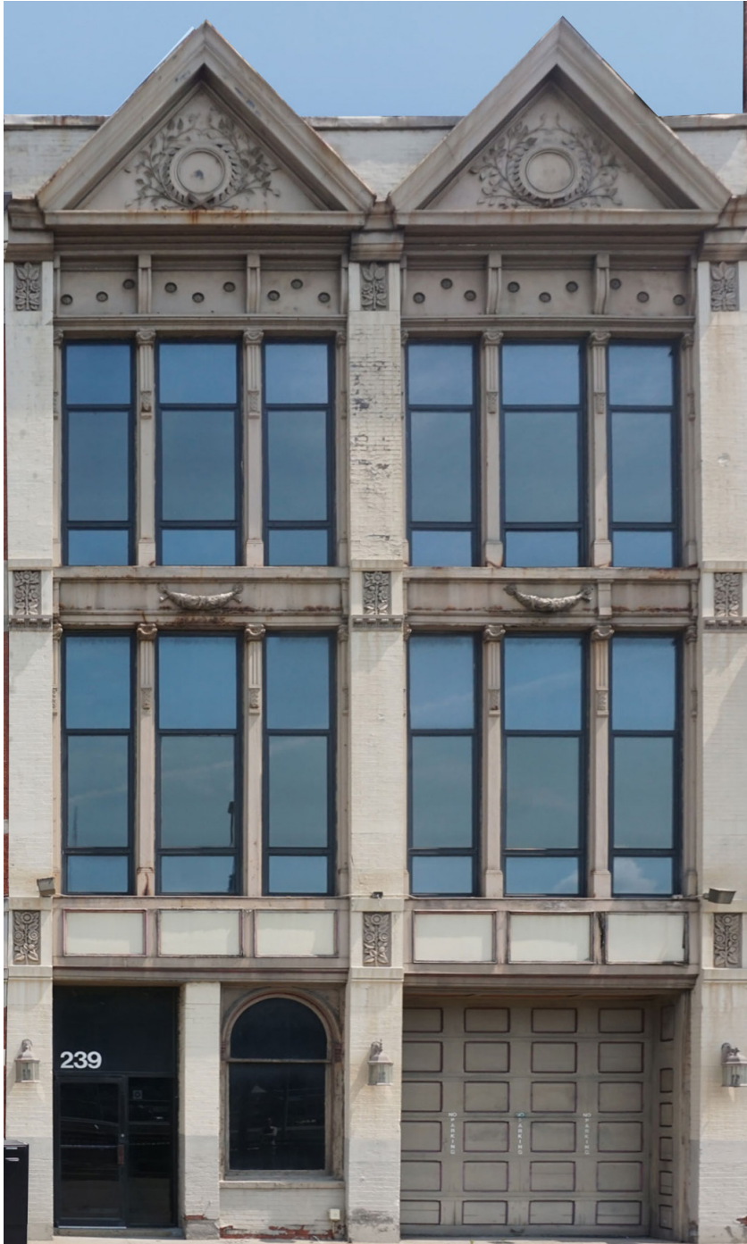
239 Fort Pitt Blvd Existing
