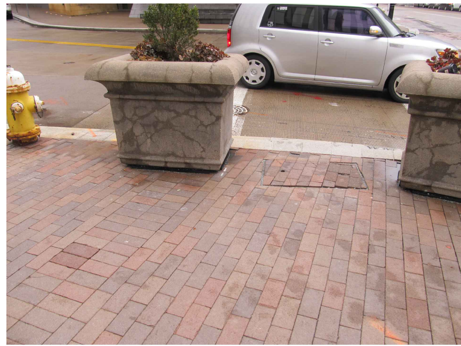
4 TRAFFIC SIGNAL ACCESS PANEL
