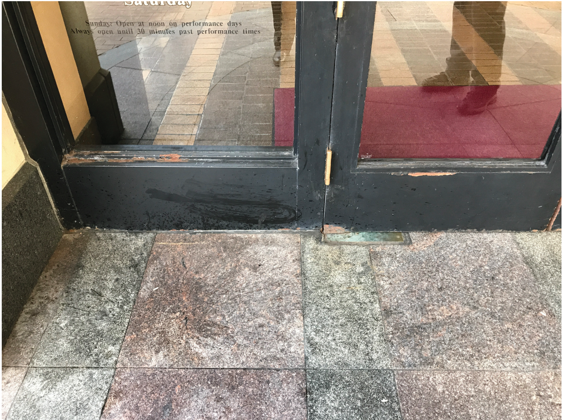
EXISTING ENTRANCE DOOR DETERIORATED CONDITION
