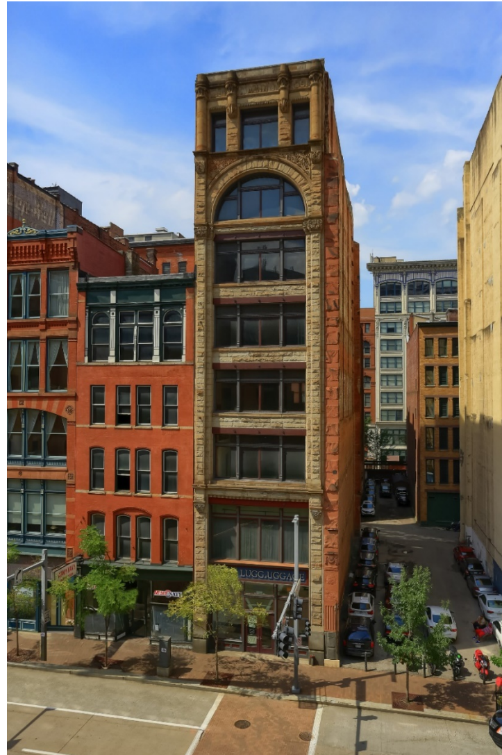
LIBERTY AVE ELEVATION SOUTH: EXISTING WINDOWS
