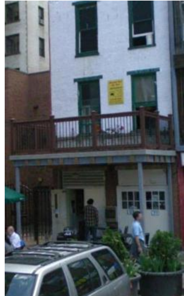
A) Market Square before 2009 renovation of $5 M
